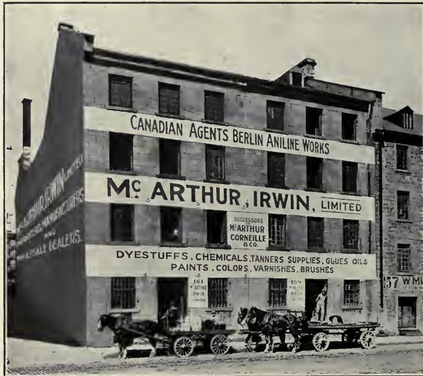
McARTHUR-IRWIN LIMITED, Factory and Warehouse, 159 to 161 Commissioners Street.
